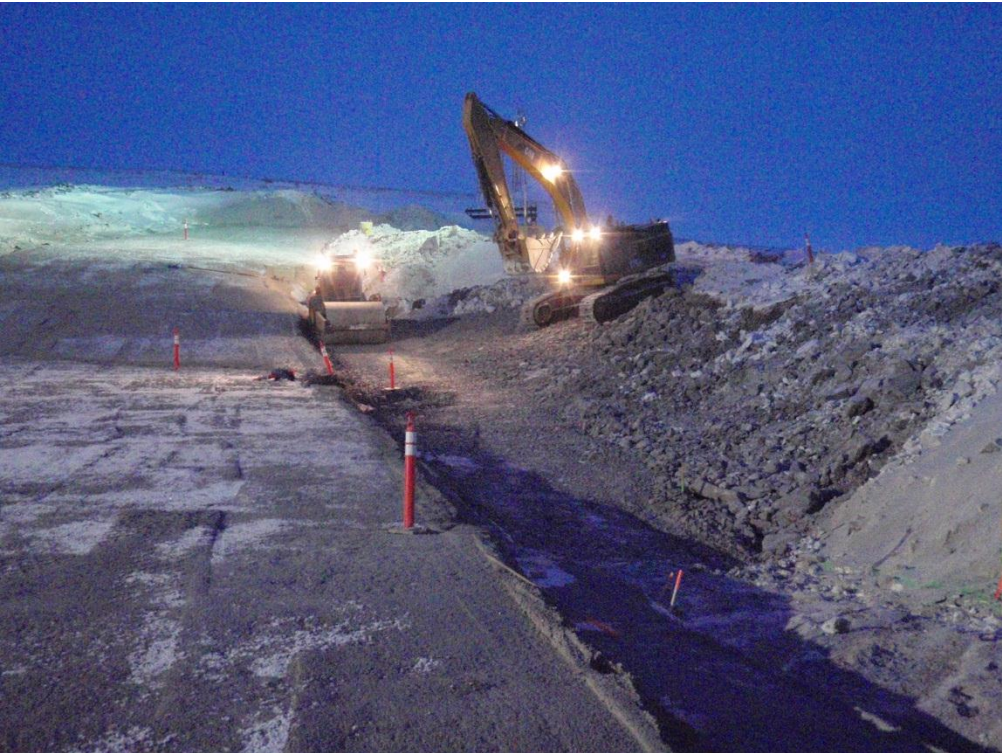
Photo 13: ~WNW of excavator and vibrator compactor working on placing and compacting material on the downstream around station 0+70 to 1+00.
