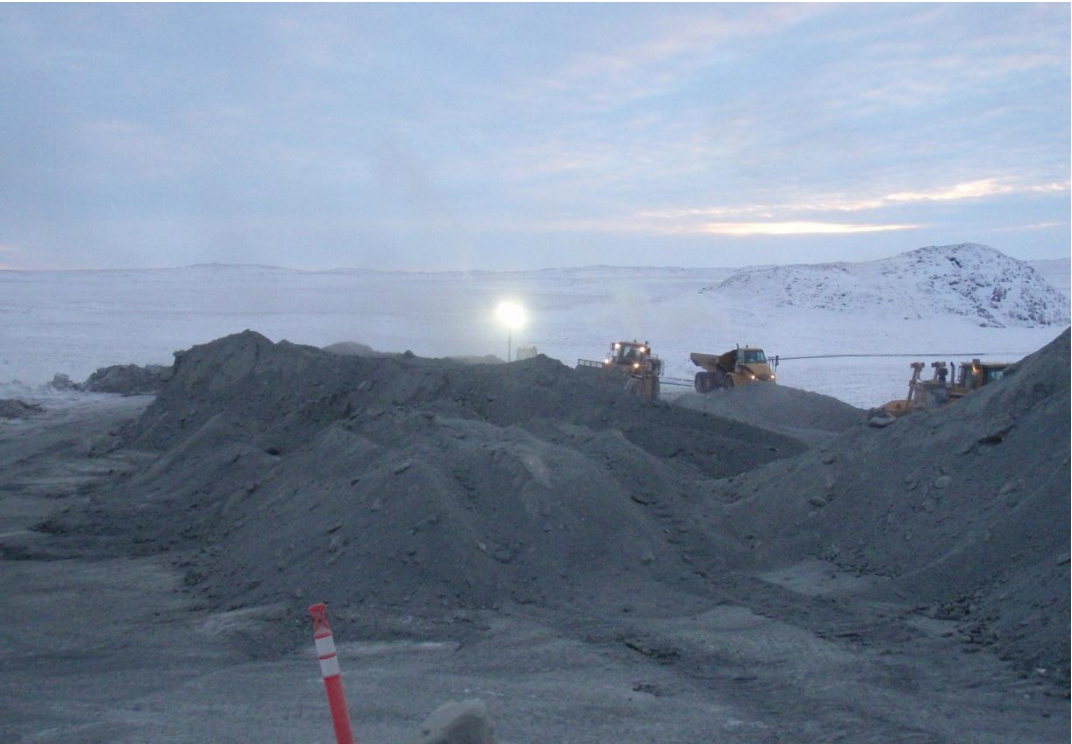
Photo 2: ~ SEE view of work on FCM stockpile at the FCP Pad. Note the equipment breaking up the large frozen lump and hauling away the frozen lumps that are unable to be broken up.
