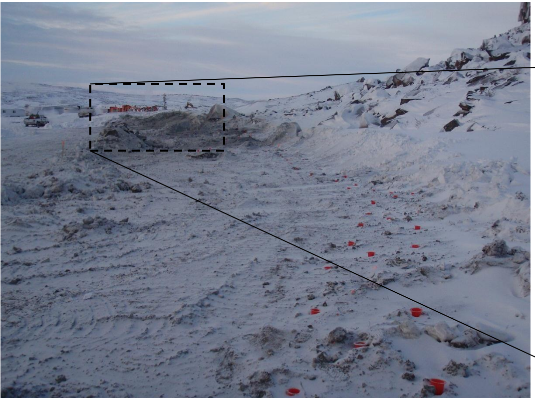
Photo 2: ~ SEE view of work on FCM stockpile at the FCP Pad. Note the equipment breaking up the large frozen lump and hauling away the frozen lumps that are unable to be broken up.
