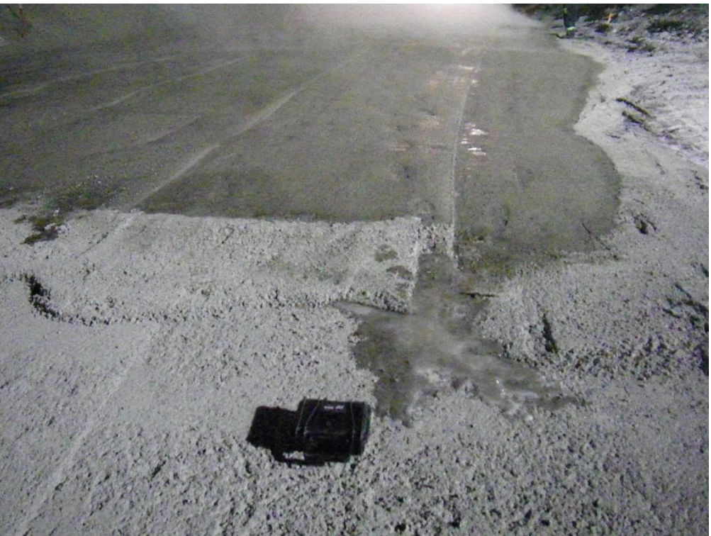
Photo 16: Water was noted to be bleeding from the end of the placed material. This photo was taken when the bleeding was first noted; additional bleeding occurred after this photo was taken.
