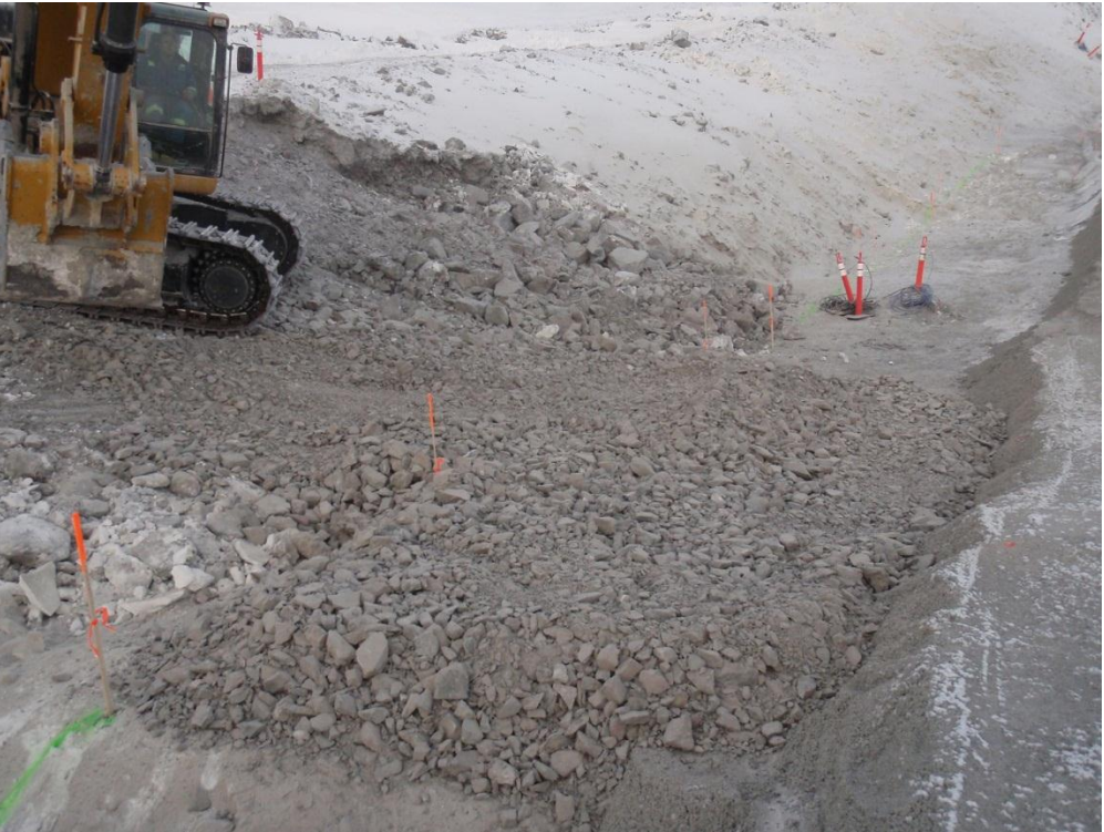
Photo 12: ~ ENE view of the 345 excavator spreading transition material around station 0+70 on the downstream.
