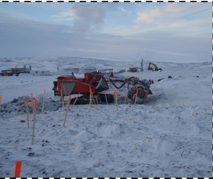
Photo 6: ~ W of the Westarc drill working on drilling the bedrock outcrop near the central east portion of the Diversion berm alignment.
