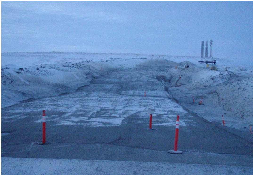
Photo 1: ~WSW view down key trench of FCM placed on 2012/ 01/ 02.
